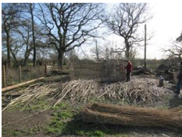
Starting from the ground with piles of hazel rods
