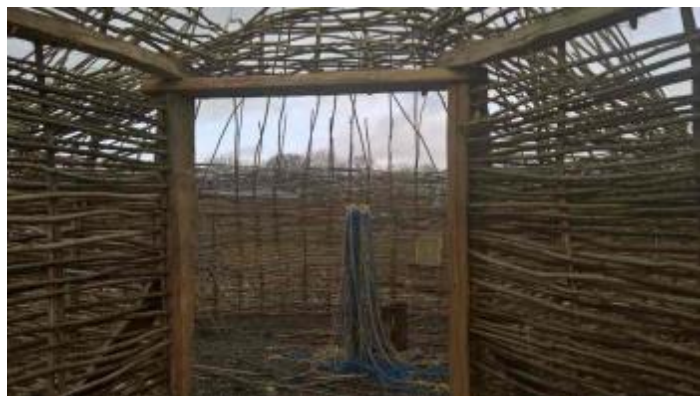
Round house creeping higher and it even has its own windows and a little porch, which like the original, is built of timbers and posts.
