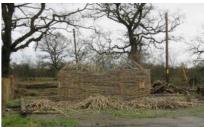
Straightening the walls and adjusting the roof
