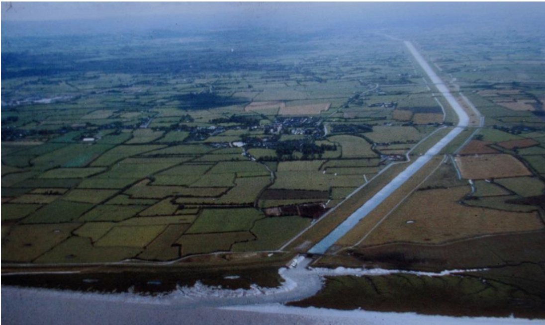
Huntspill Sluice at the river's western end separates the river from the River Parret. Courtesy SWHT
