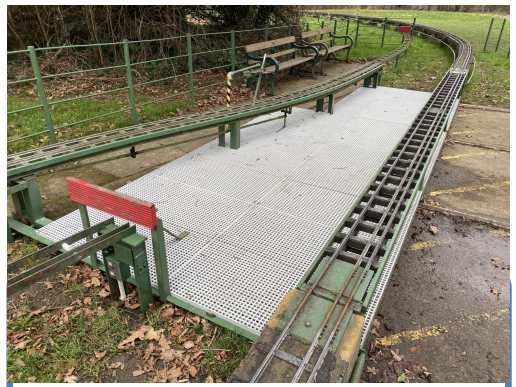
New deck fitted to traverser
