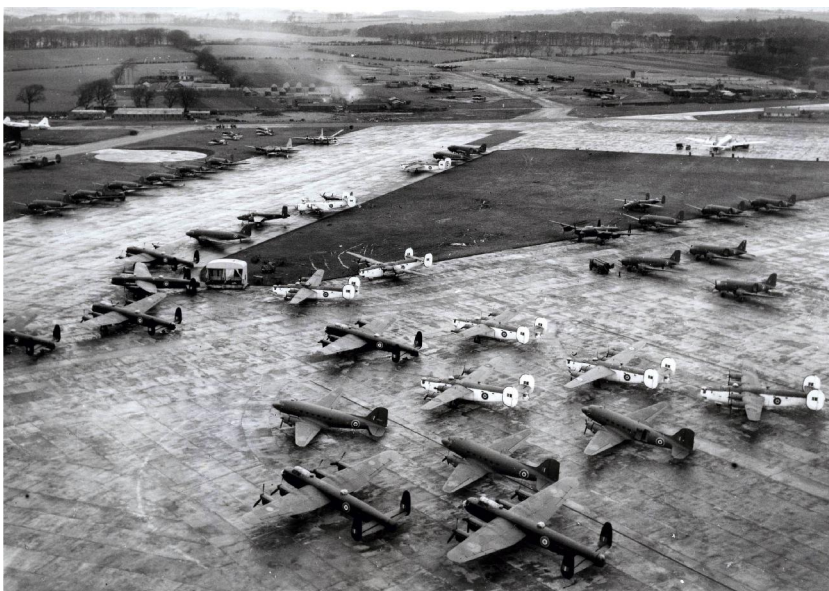
c.1944 - The second world war brought remarkable change and challenge to SAL. The Palace of Engineering was hastily relocated to its present location from Bellahouston Park in Glasgow, tarmac runways were laid and SAL became the reception organisation for hundreds of aircraft built in the USA and Canada. This remarkable view shows B-24s, B-25s, B-17s, C-47s, a solitary C-54 along with many Canadian manufactured Avro Lancasters and probably others. Trans-Atlantic movements on this scale demanded the provision of an air traffic control service, and this remains at Prestwick to this day. (via Dugald Cameron)
