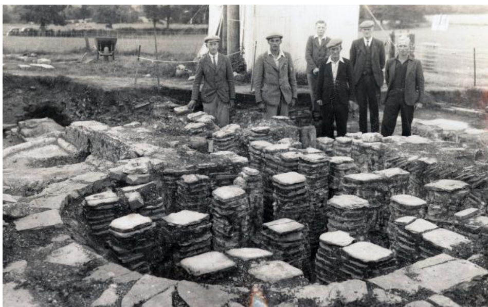
Image showing the pilae which supported the hypocaust floor at Low Ham, 1940s excavation.
