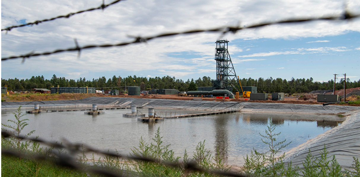
Evaporation pond at Canyon Mine. Blake McCord
