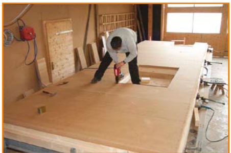
The large majority of panel elements can be prefabricated, unaffected by weather conditions
