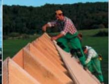
Tongue and groove edges and low weight make for easy use.
