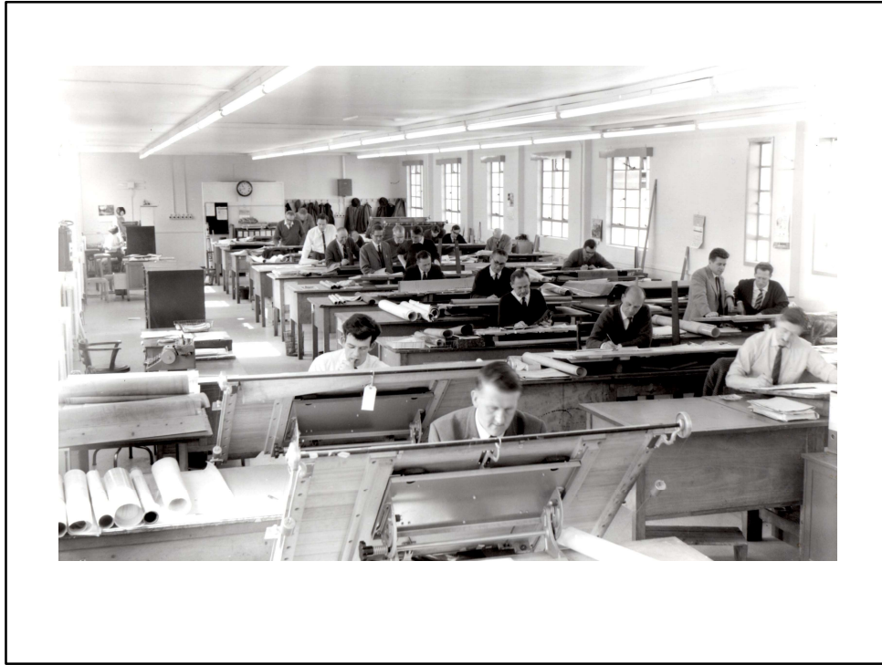
This was our design department in the 1970's. We were drawing with pencils and pens on paper, linen and plastic sheets supported mainly on flat drawing boards.
