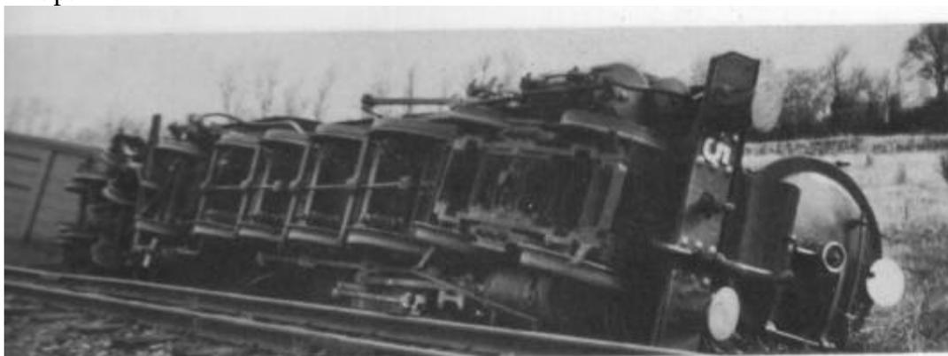
Underside of 4-8-2 Hercules, as revealed after the leading van in the train was blown over in a gale, dragging the tender and then the engine over with it. Well visible are the helical springs of the coupled boxes, and the brake cross and central pull rods.
